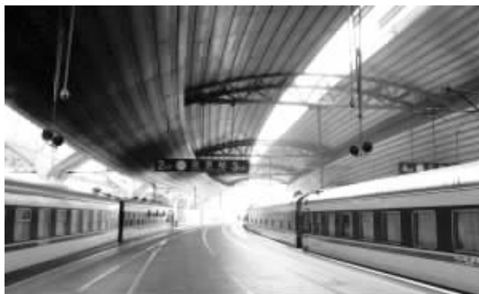
Figure 2-2 The platform of Beijing Railway Station
